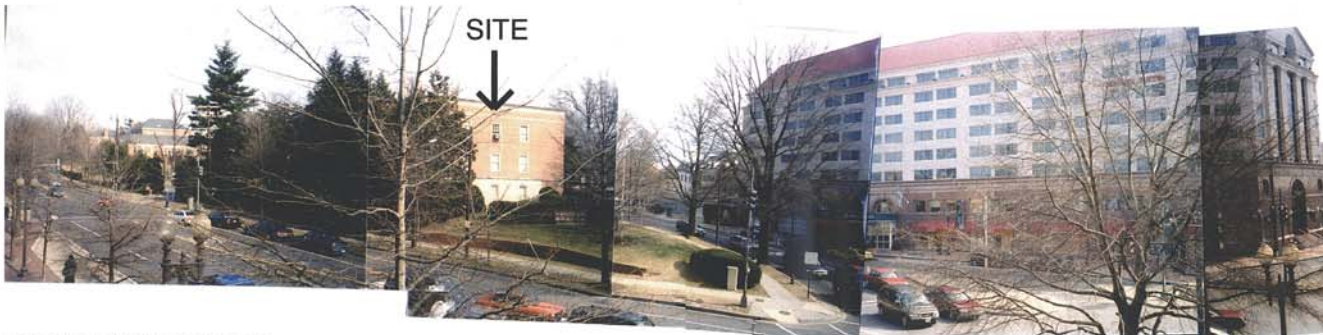
3. VIEW OF SITE LOOKING EAST
